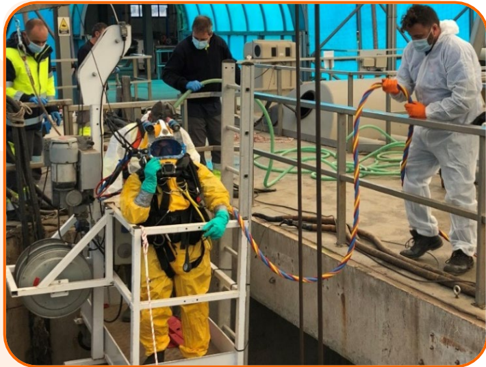
Works in contaminated waters
