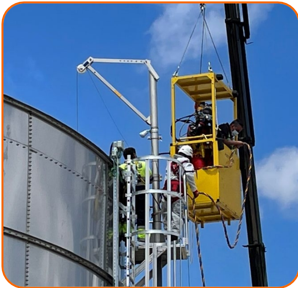
Underwater maintenance of water tanks in treatment plants
