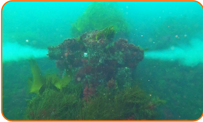
Underwater inspection and maintenance of outfalls and inmissaries
